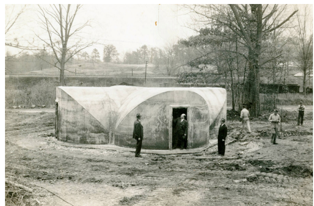
Figure 2. The Clover aka the Igloo - Experimental concrete housing in Vicksburg, Mississippi. February 1944. Image courtesy of LeTourneau University Archives.
