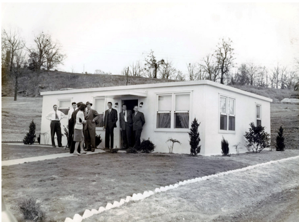
Figure 3. The first Tournalaid house was poured in Vicksburg, Mississippi in November 1945. Image from the in-house publication NOW. March 15, 1946. Vol 10, No.44.
